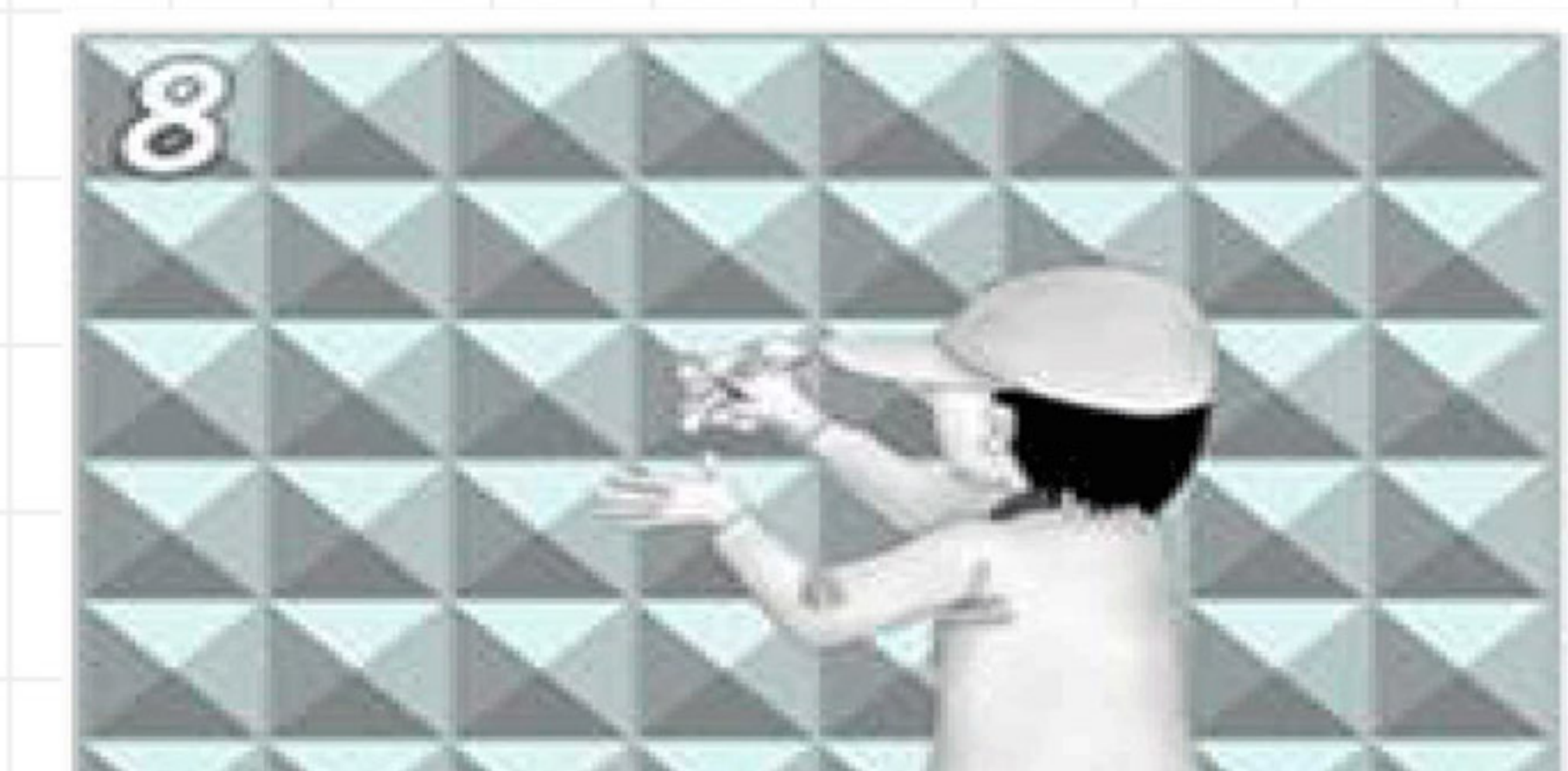
8. Clean the wall surface
