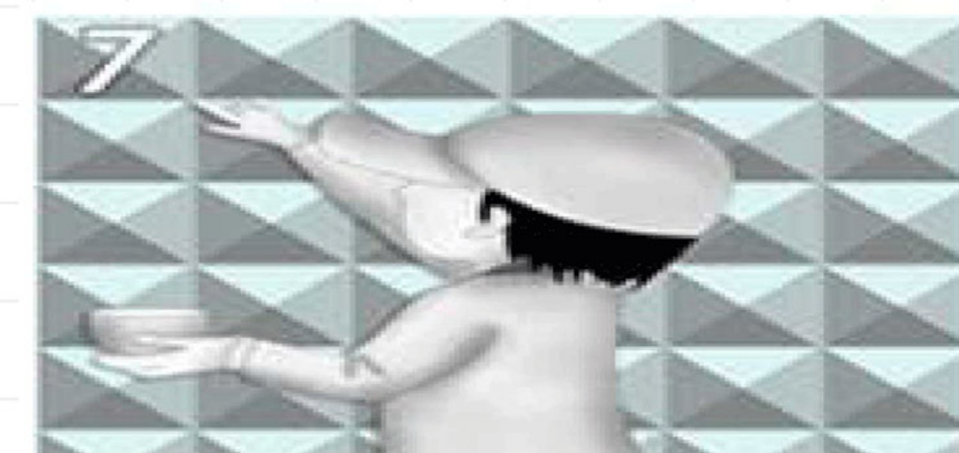
7. Using fillers to fill the gap between two panel
